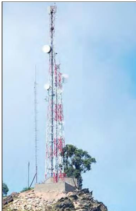
Safaricom is migrating its TDM mobile backhaul sites, such as Lewa, Kenya, (above) to the Eclipse Packet Node hybrid microwave radio platform to support 3G and WiMAX data growth on Ethernet while preserving sufficient E1 capacity for 2G and 3G voice.
